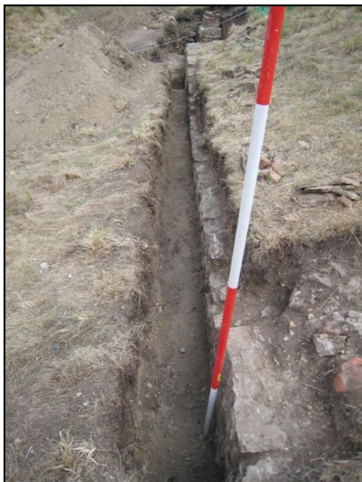
Fig 3 The unbroken inside face of the south house wall, looking east from the estimated mid-point
